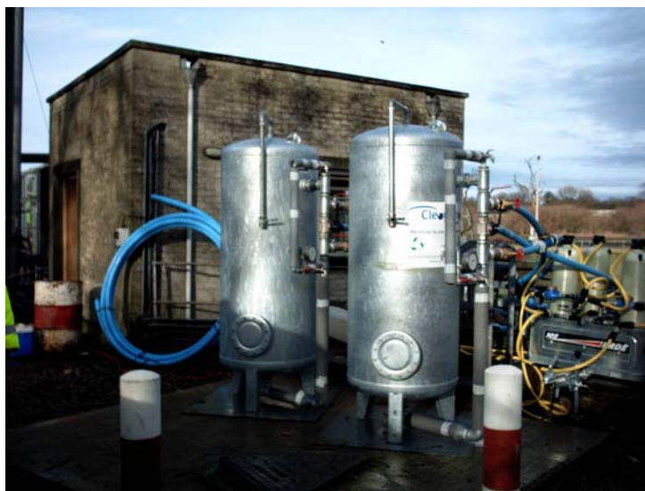
Figure 10. The two full-scale filters at Malton WwTw, one packed with sand medium the other with medium grade glass
